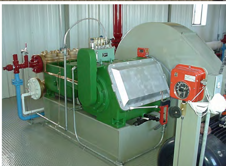
20'x45' portable waterflood station.
