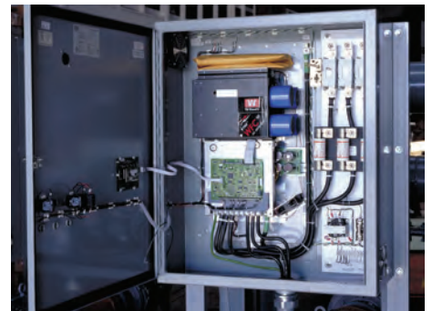
100 HP electric motors with TB Woods AC inverters.
