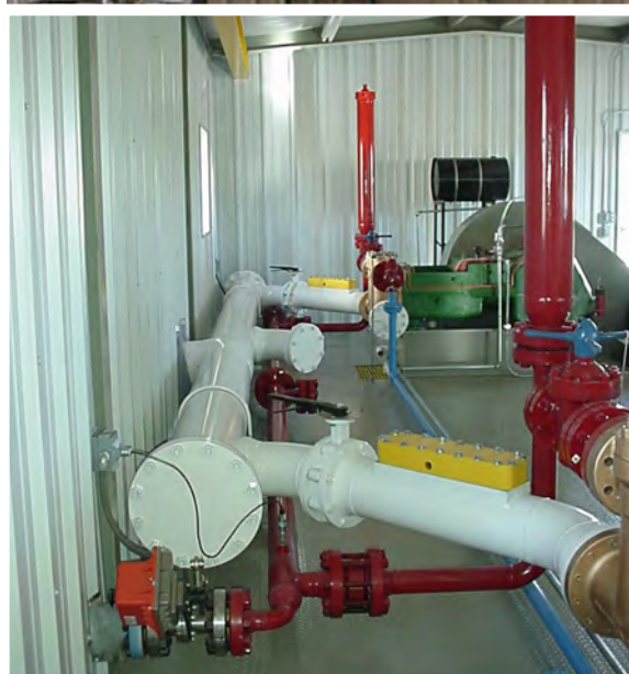
20'x45' portable waterflood station.
