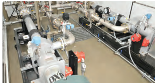
Water Transfer Skid
