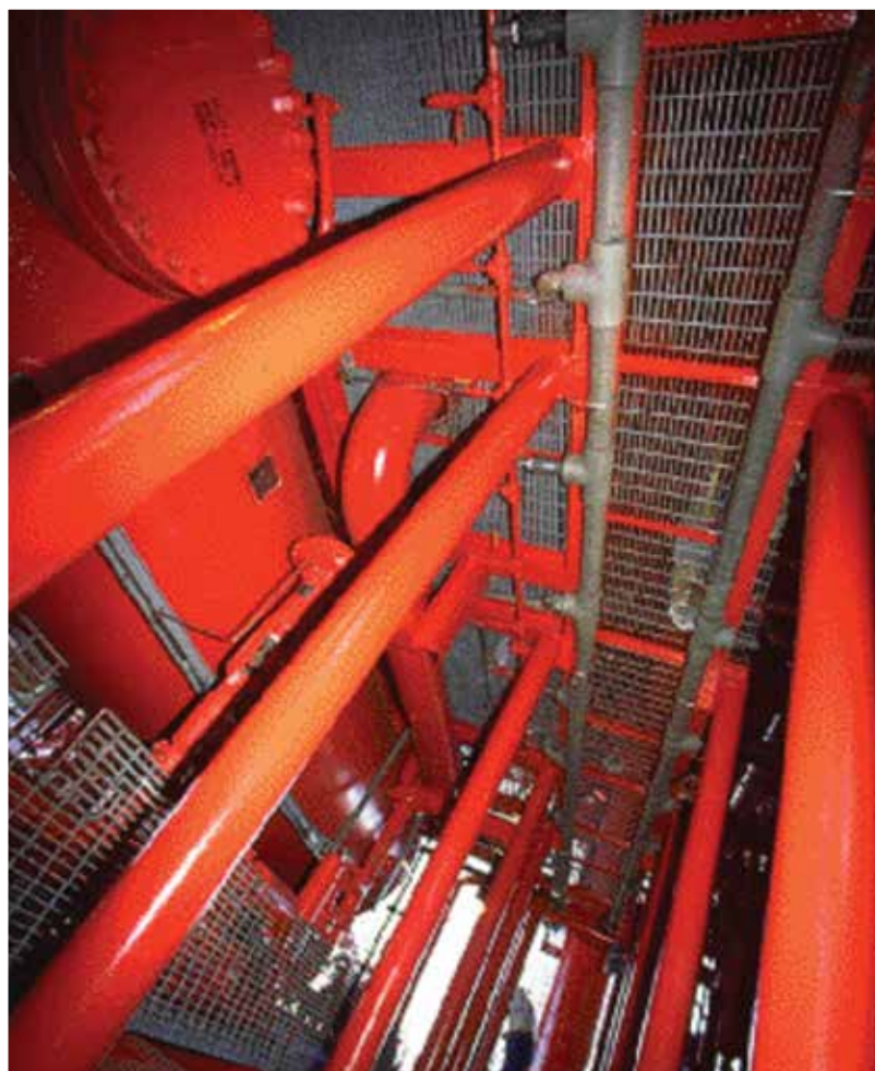
Typical offshore application: Fire Protection Deluge System, 2,000M-FP.
