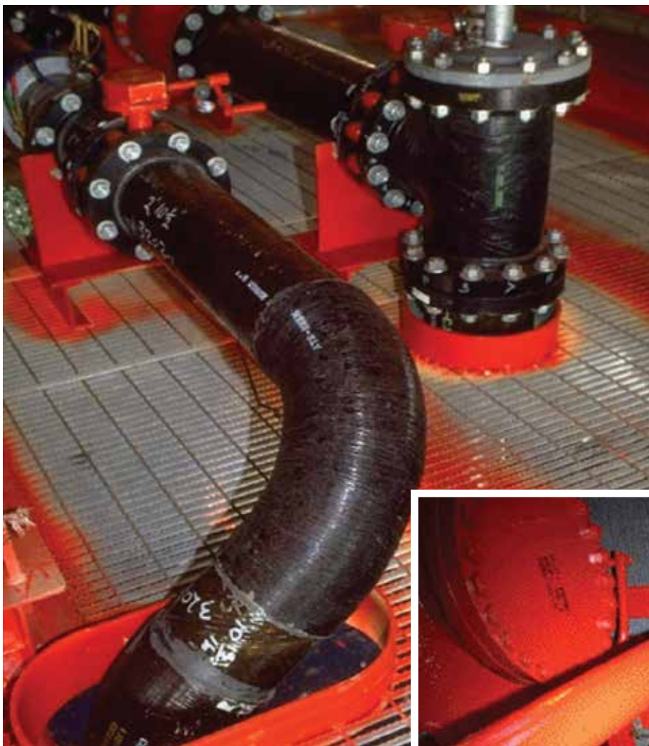
Wet fire water 2,000M. First platform to install FRP in Deluge System in the Americas.
