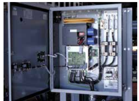
100 HP electric motors with TB Woods AC inverters.
